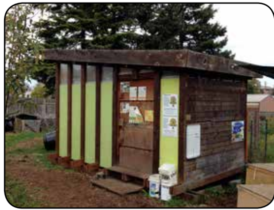
Support Existing Facilities
