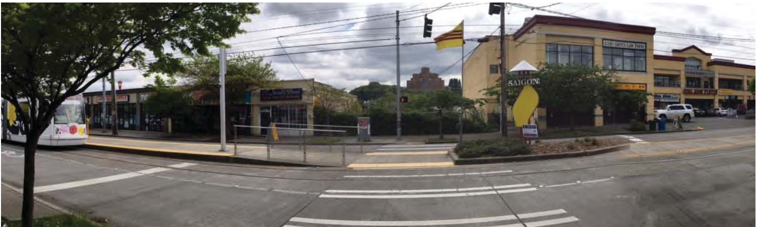
LOOKING SOUTH ACROSS SOUTH JACKSON STREET
