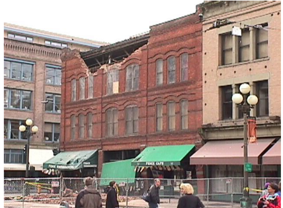
1999 Nisqually earthquake damage. USGS photo.
