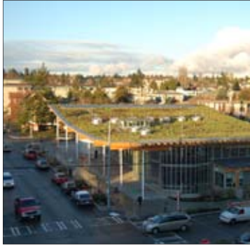
Green roof on the new Ballard library.
