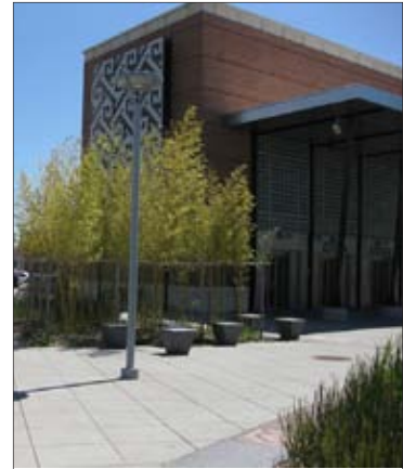
Beacon Hill LINK Light Rail Station.
