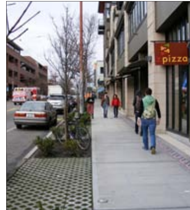
This streetscape is designed with pervious paving, street trees and other planting—types of green stormwater infrastructure.
