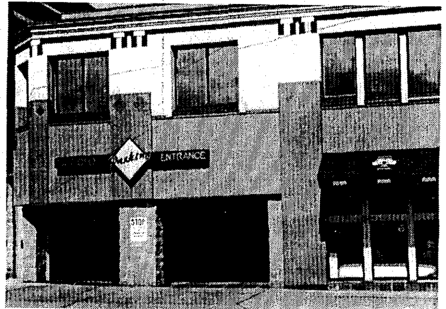
Existing parking structure on North side of Green Lake
