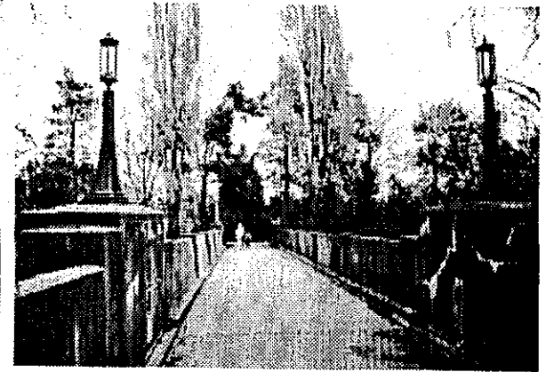
Existing bridge over Aurora Ave. N
