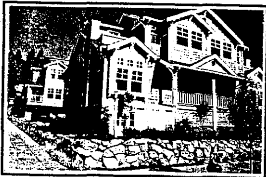
TB-7 New Residential Construction 7726 E Green Lake Dr. N
