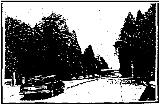
TL-8 Aurora Avenue N at Woodland Park View south with footbridges
