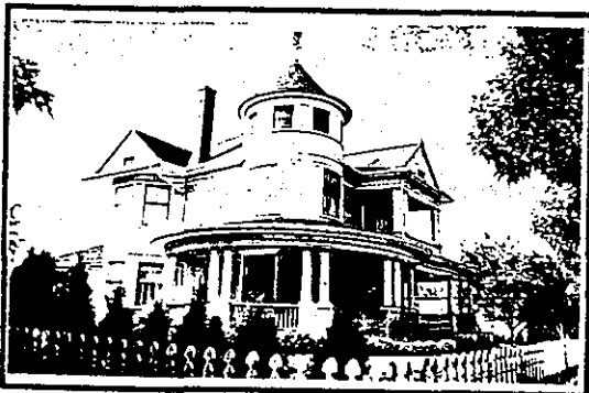
TB-5 Victorian Residence 2153 N 62nd St.
