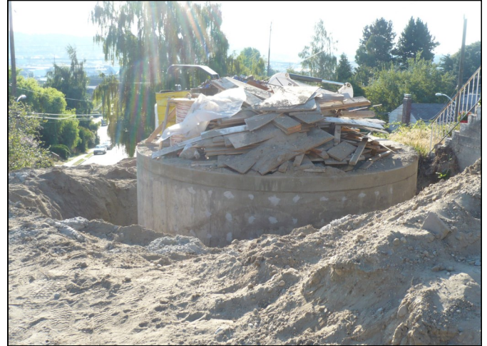
Major grading work at Hazel Heights
