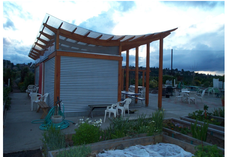
Interbay's shed needed a permit
