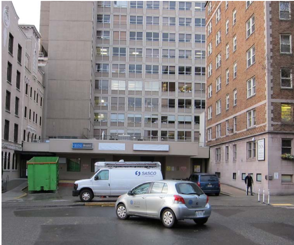
View of Terry Avenue, looking north - existing condition.
