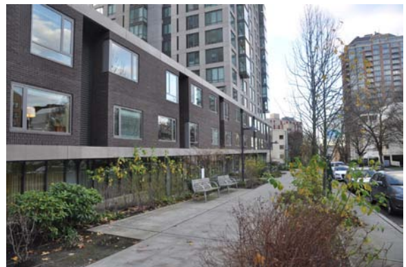
Along Ninth Avenue, the massing is lower in scale and horizontal.
