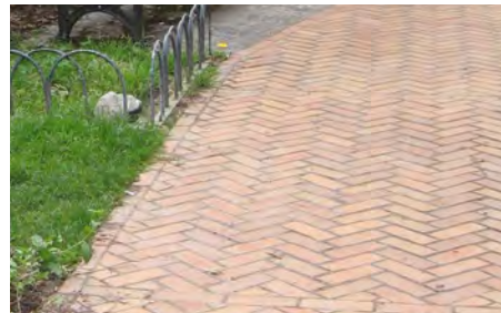
Existing and Reclaimed Brick Paving
