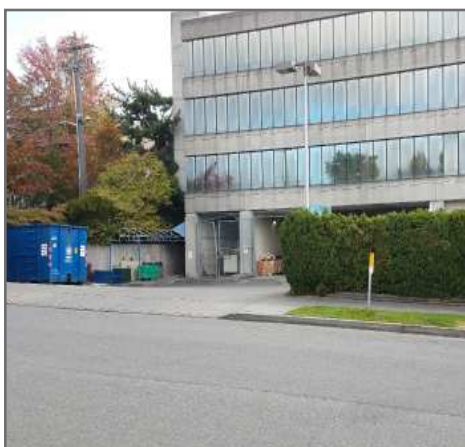
Photo: Service entry on 16th Ave.
