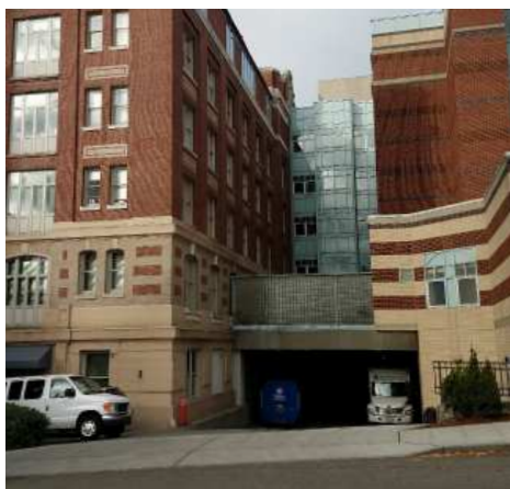
Photo: Service entry on 18th Ave.
