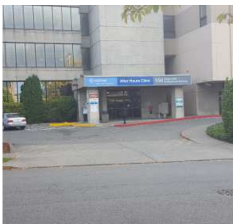
Photo: ED/ After Hours Clinic Entry Drive
