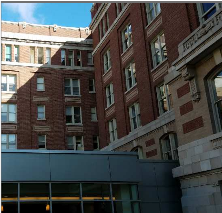
Photo: New construction meets old structures at Swedish Cherry Hill.
