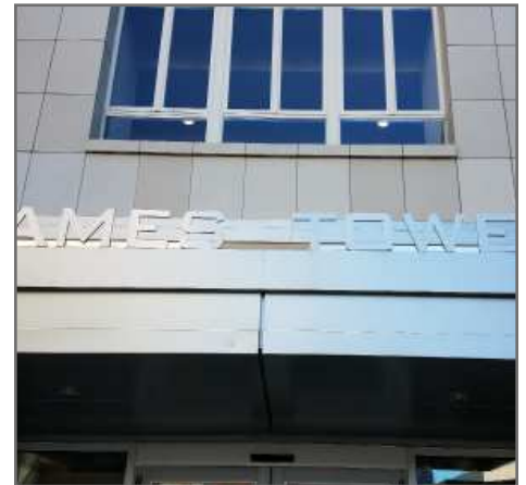
Photo: Existing James Tower facade detail.
