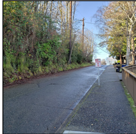
9 Widening of Dravus St
