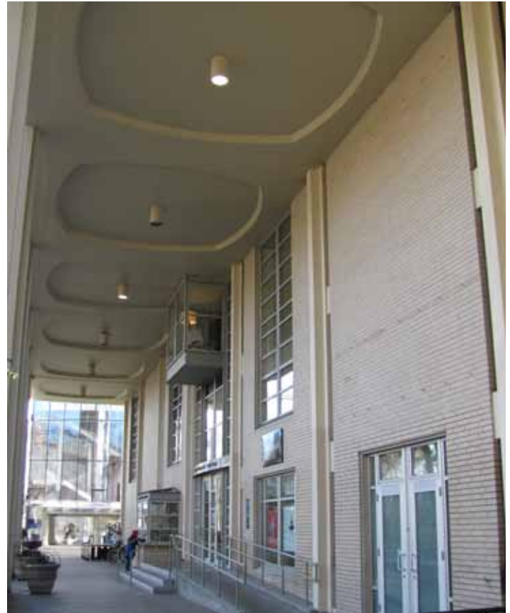
Left: 2013 detail of colonnade concrete post base in the Playhouse courtyard. Source: Artifacts Consulting, Inc.
