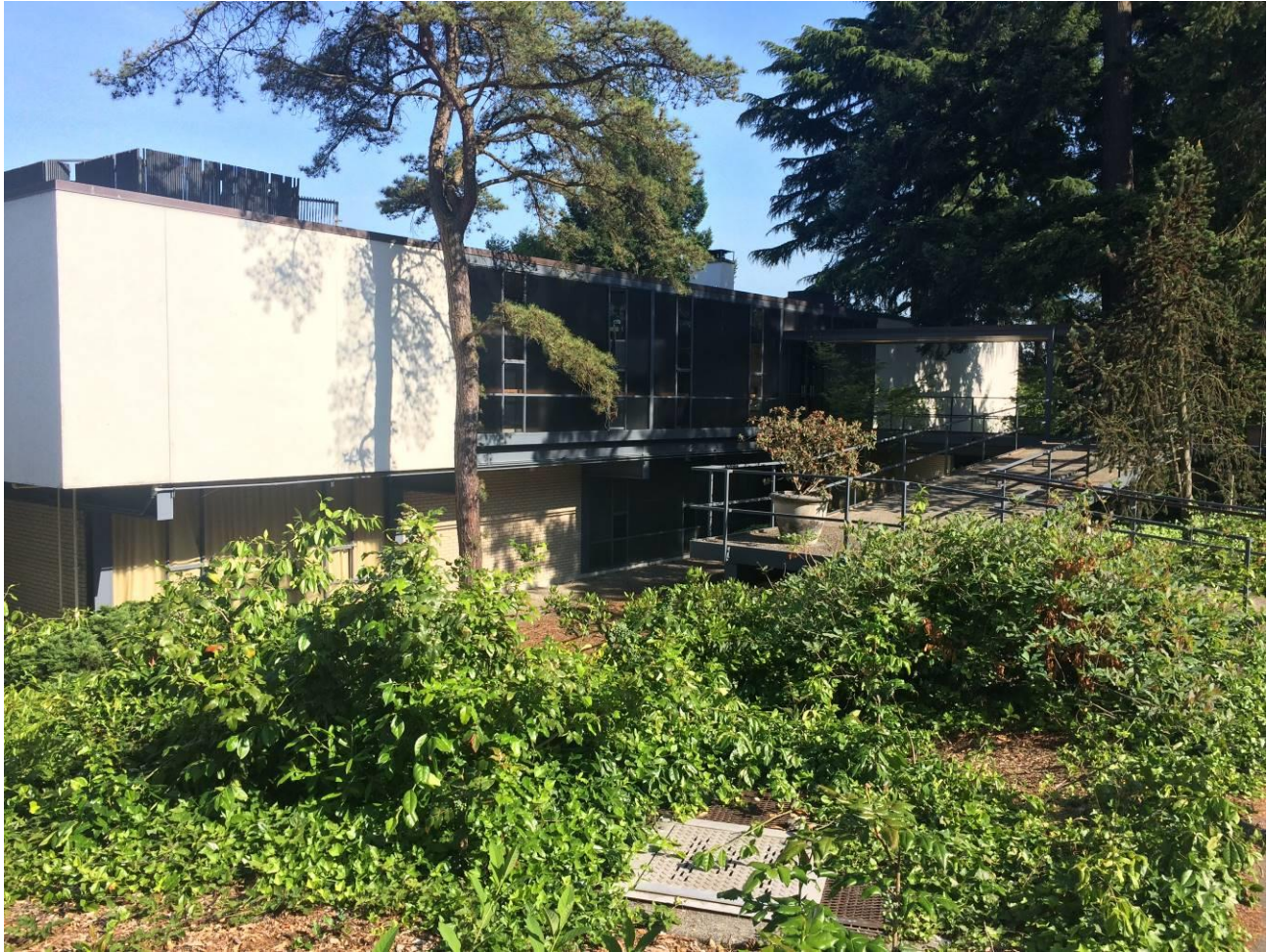
Figure 39. Above, looking southeast at the primary west facade and entry ramp.
