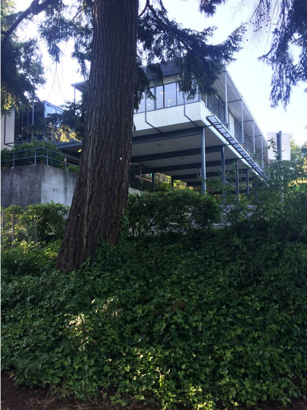
Figure 43. Above, looking northwest at the western portion of the south facade and the dining room section of the building above the lower parking lot.
