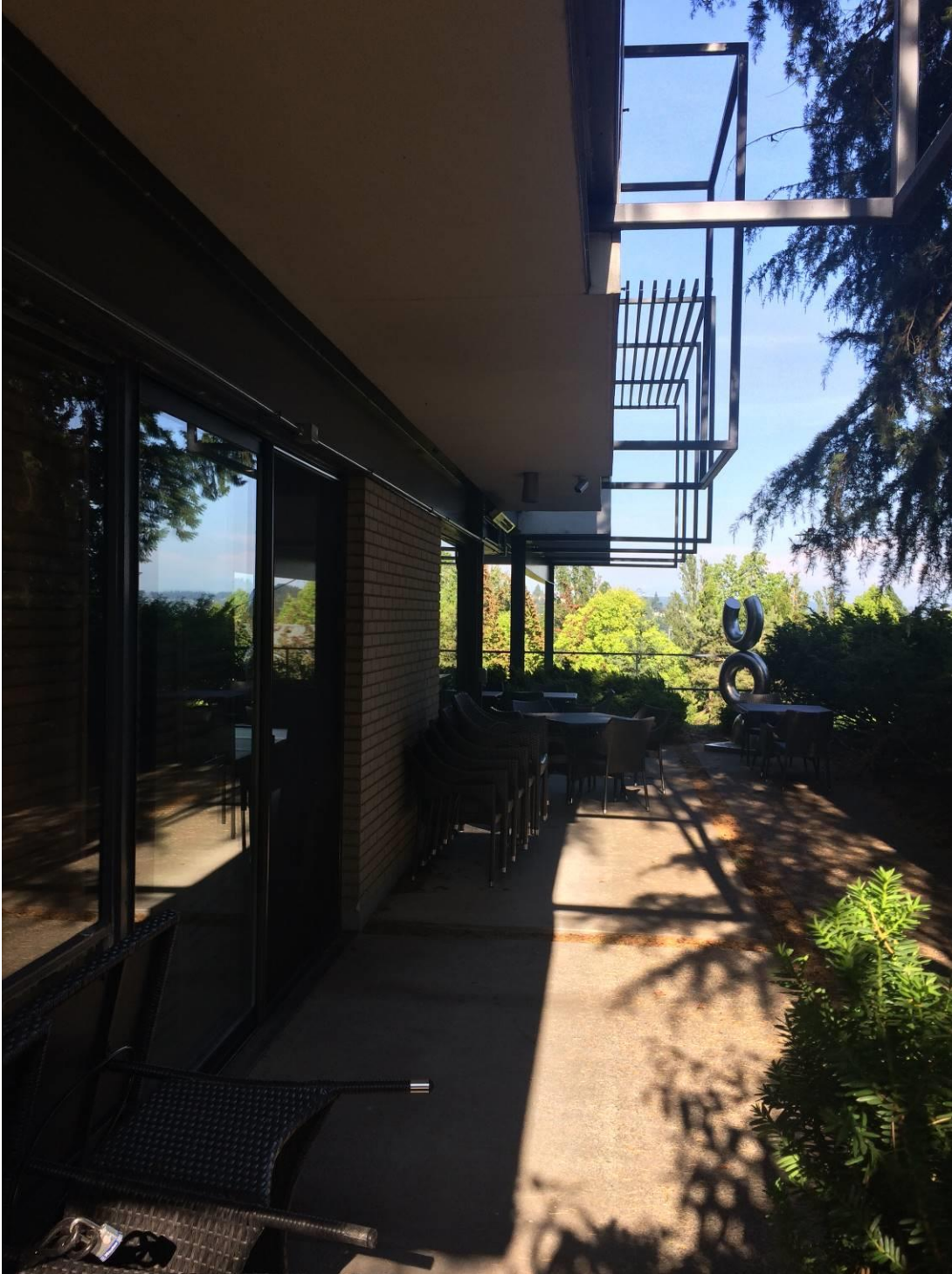
Figure 57. Looking east along the south perimeter all at the lower (first) floor terrace.
