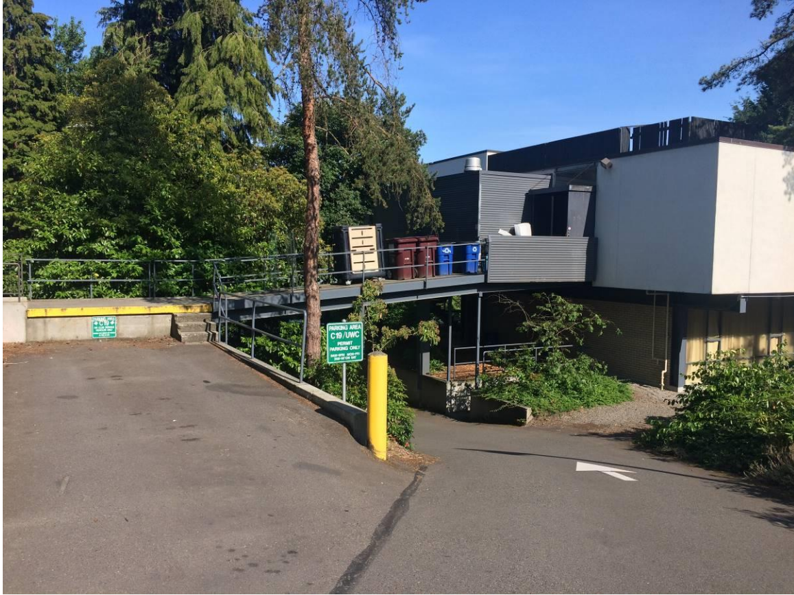
Figure 42. Above, looking southeast at the entry drive, partial north facade and service walkway. The grey metal clad walls enclose an expansion of kitchen service spaces.
