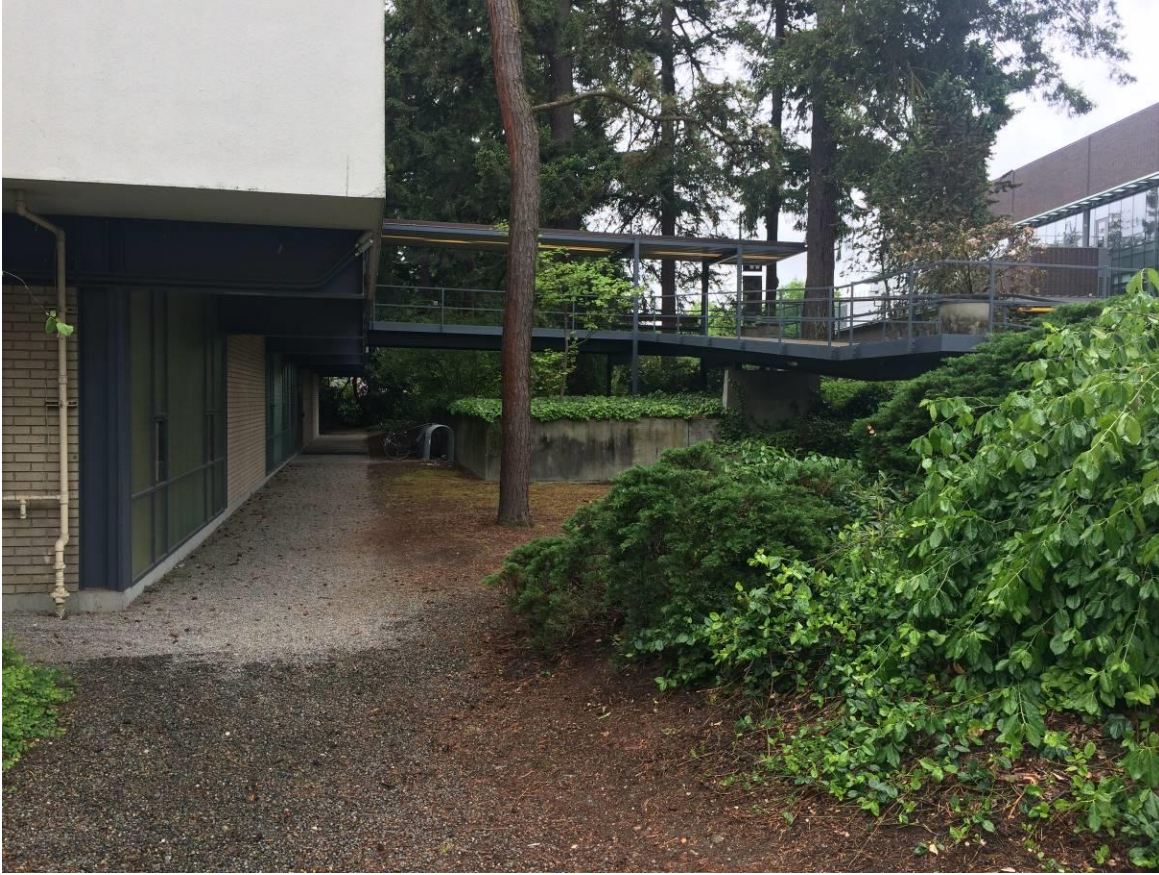
Figure 58. Above, looking south at the landscape front yard (west) and grade at the lower (first) floor.
