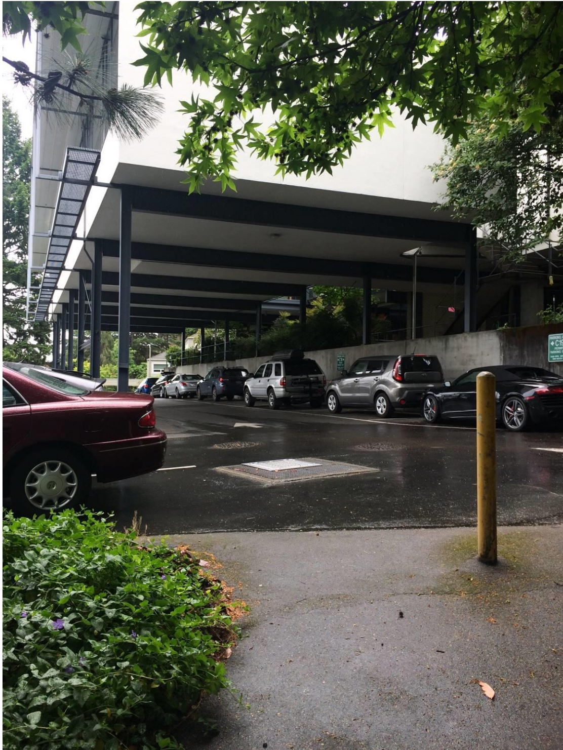
Figure 60. Looking southwest in the parking lot below the upper floor and the building's steel frame. The retaining wall visible on the right supports the grade at the lower (first) floor.
