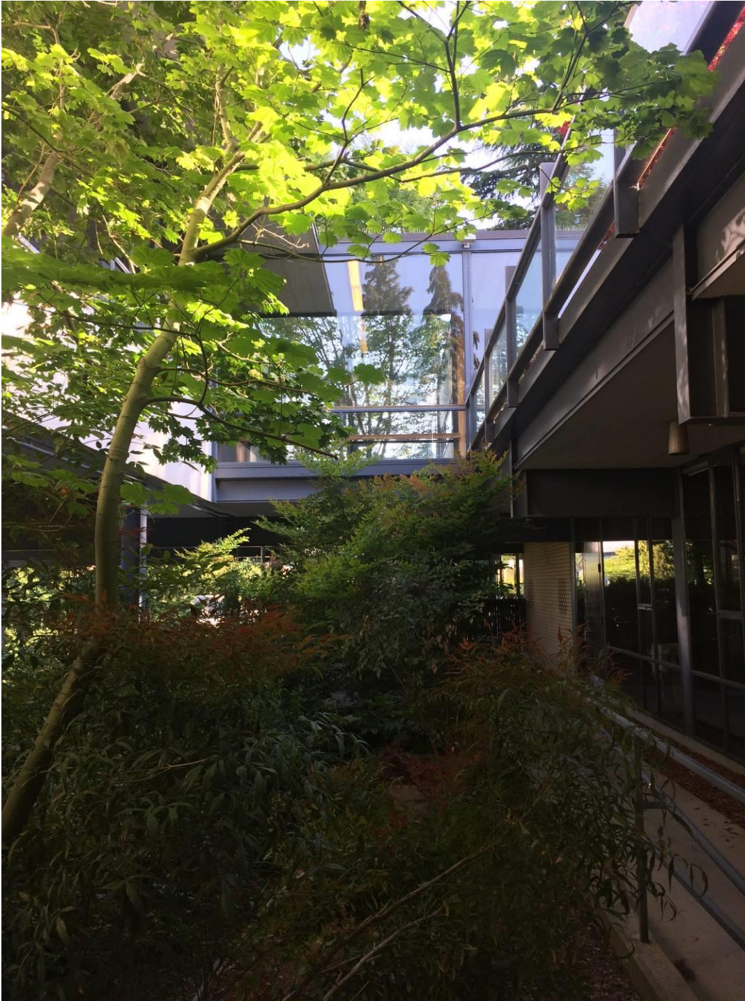
Figure 56. Looking south in the lightwell between the dining room (left) and central courtyard (right), with the upper (second) floor south corridor in the background.
