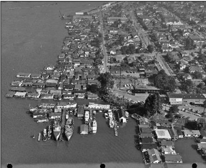
Figures 11 and 12. Top and above, aerial views of the Lake Union shoreline and portions of the Eastlake neighborhood near Fairview Avenue East and East Newton Street in 1962. The area still contained a mix of residences, modest houseboats, marine-related industrial facilities, such as the Lake Union Dry Dock, and low-scale commercial buildings. (Seattle Municipal Archives, above 63791, and below 63787)
