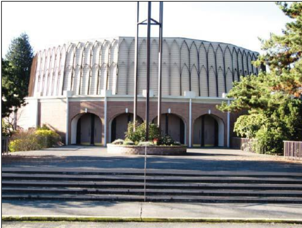
Figure 44 , below, Glendale Evangelical Lutheran Church (1967), Burien.
