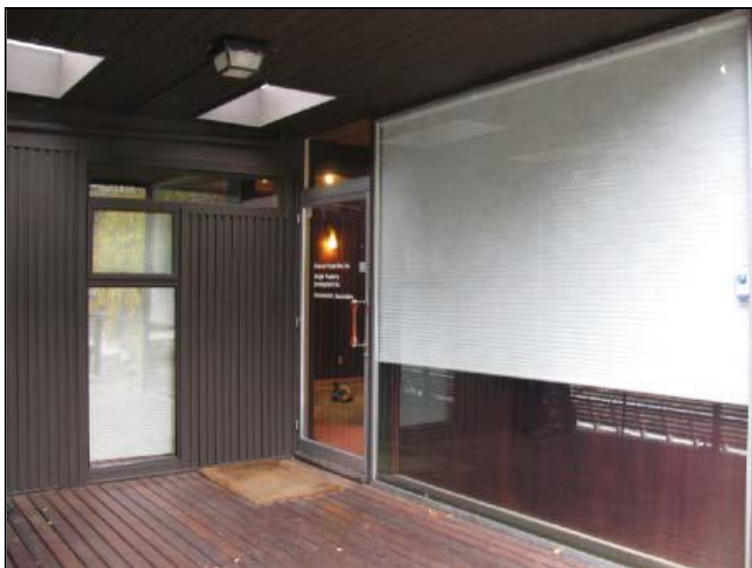
Figures 38 & 39. Below left, a view showing the original aluminum frame entry and window, right, and more recent infill with vertical wood strip cladding, and detail of original door pull (2009 photos).
