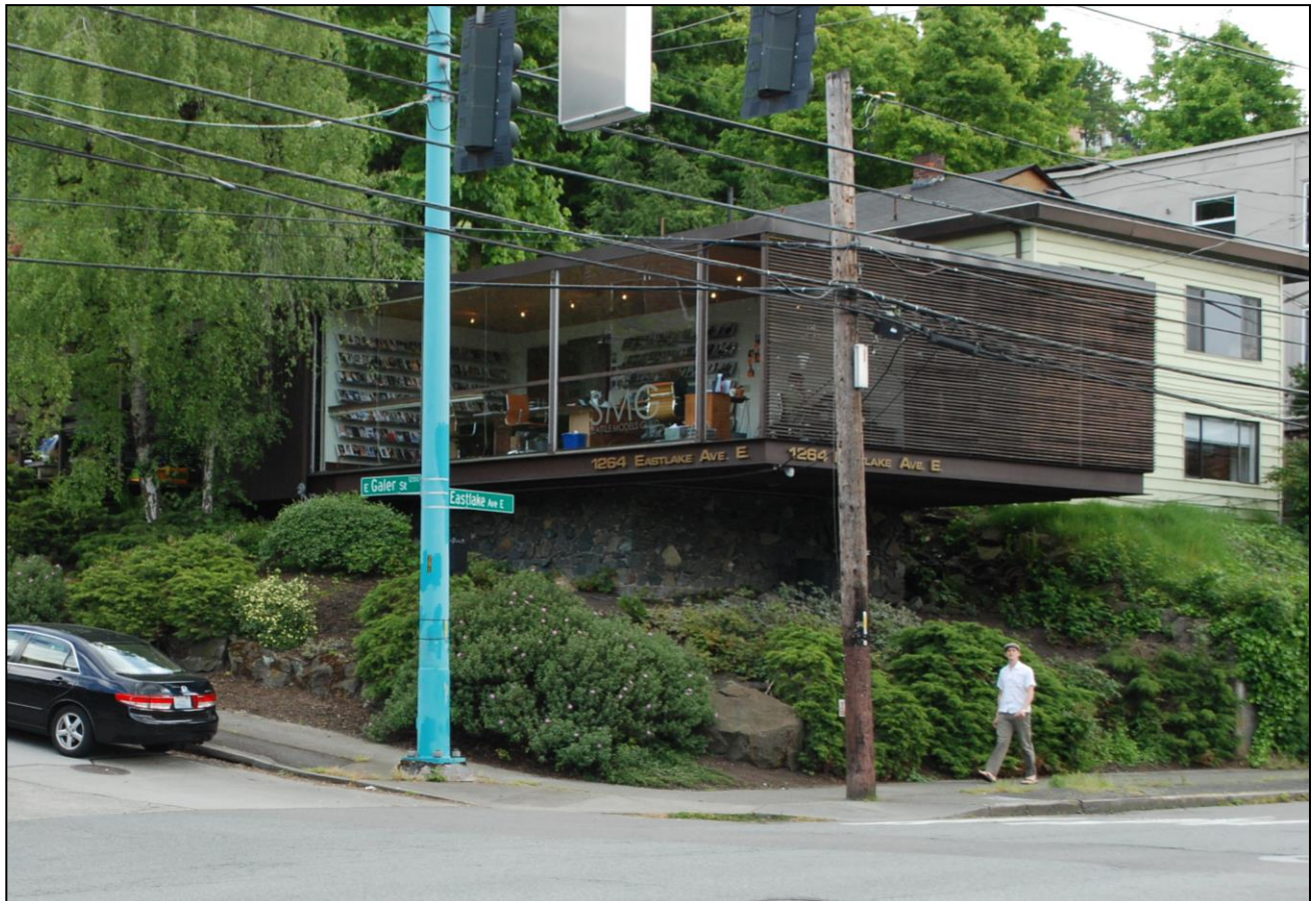
Figure 30. Below, the primary north and west facades. (2014)
