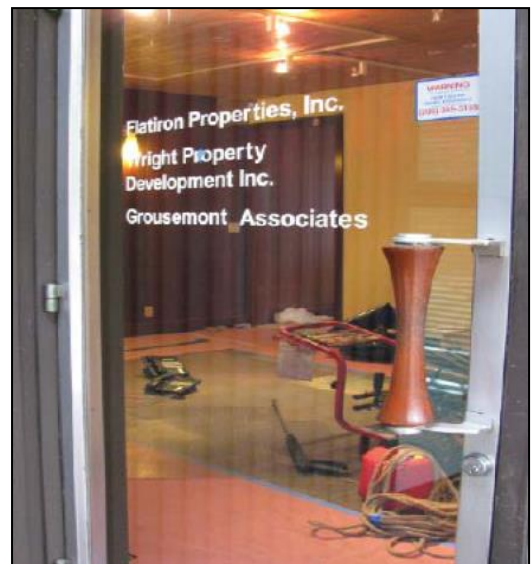
Figures 38 & 39. Below left, a view showing the original aluminum frame entry and window, right, and more recent infill with vertical wood strip cladding, and detail of original door pull (2009 photos).
