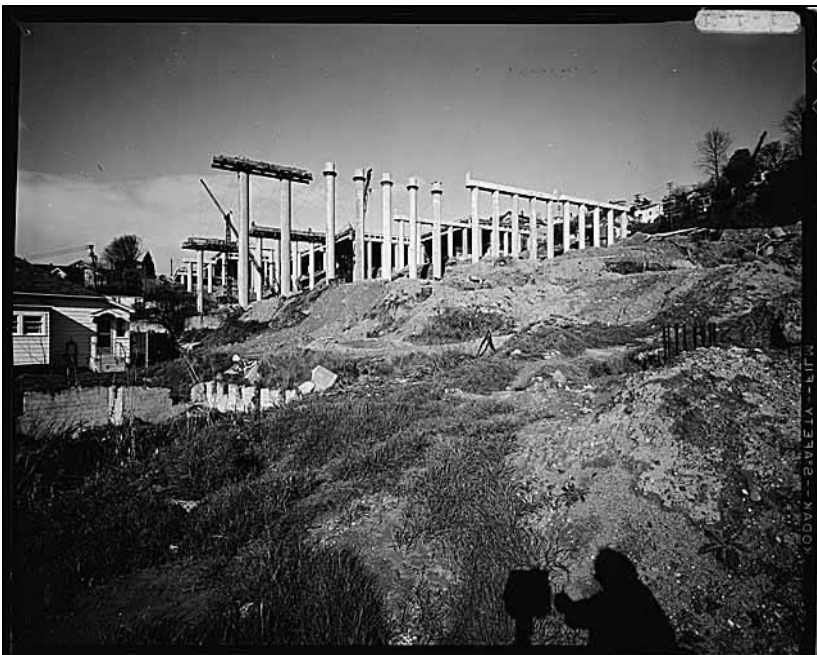
Figure 18. Below, historic photo view of construction of the I-5 highway in 1961. The tall support columns shown in this view are one block east of the subject property. (MOHAI, 1986.5.4016.1)
