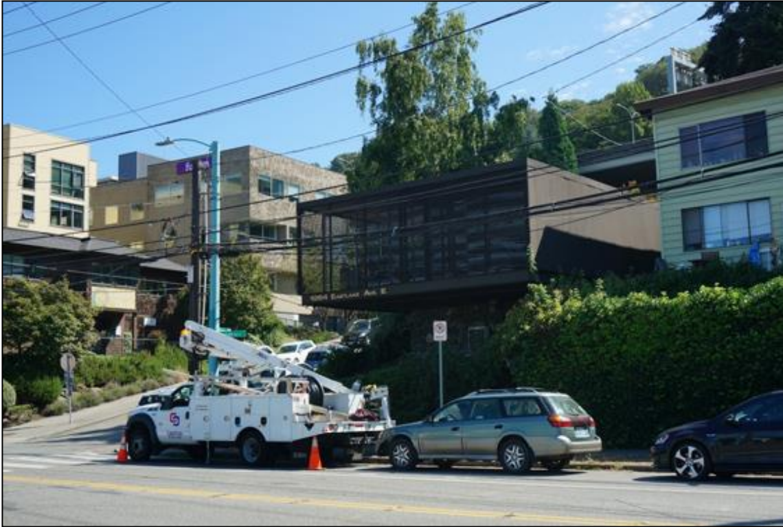
Figure 27. Above, looking northeast at the primary west façade and secondary south facade.
