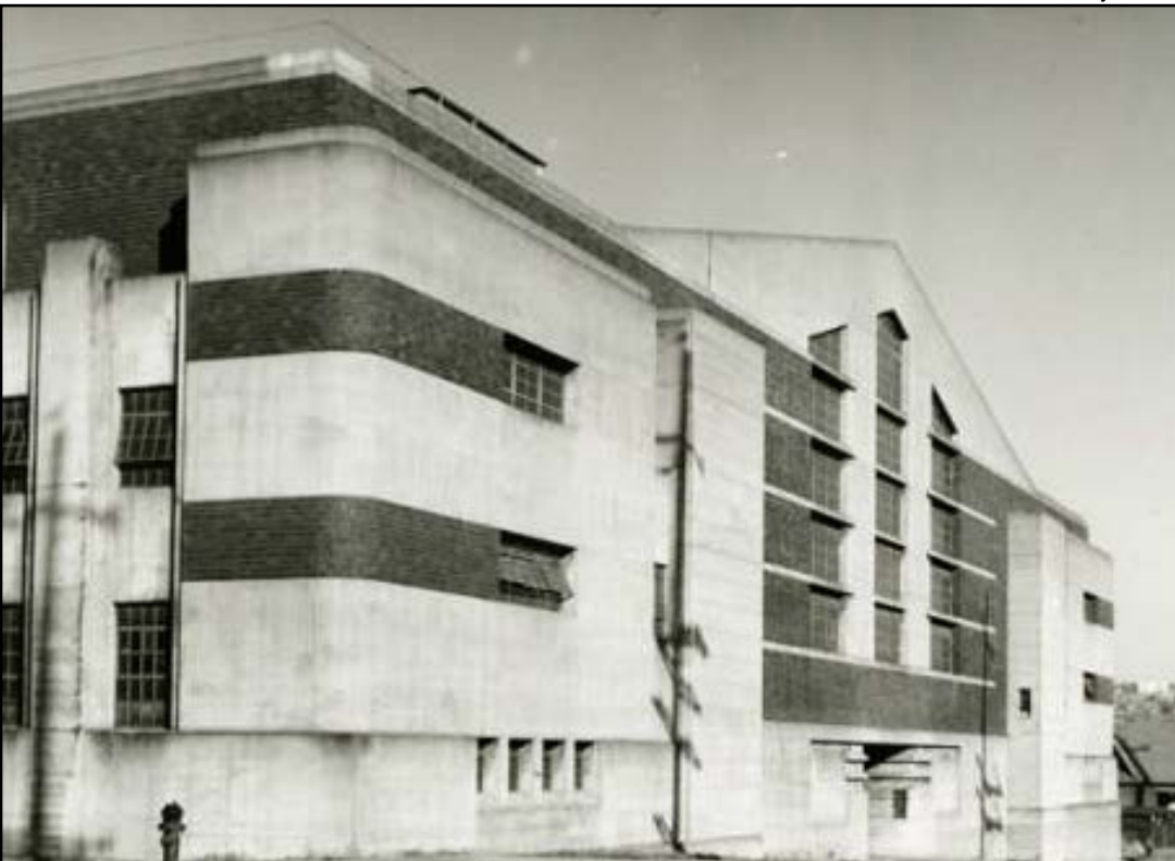
Figure 96 • Seattle Center House, 305 Harrison Street (1939, Naramore & Young, City of Seattle Landmark)
