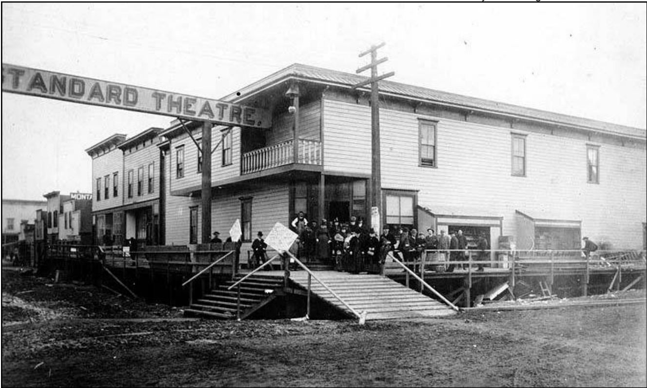
Figure 57 • The Standard Theater (formerly the Alhambra Theater, 1884) on Second Street between Washington and Main streets
