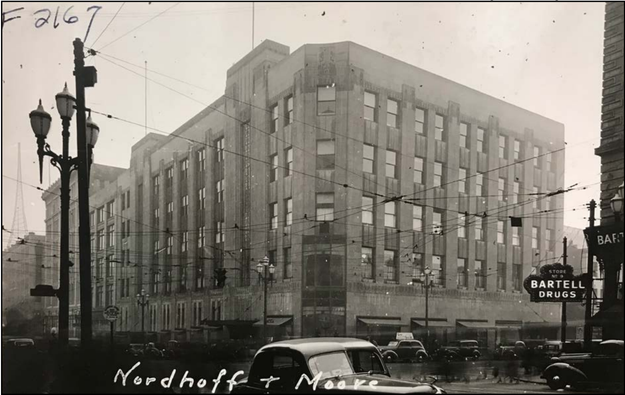
Figure 38 • J. C. Penney at Second Avenue and Pike Street, 1937
