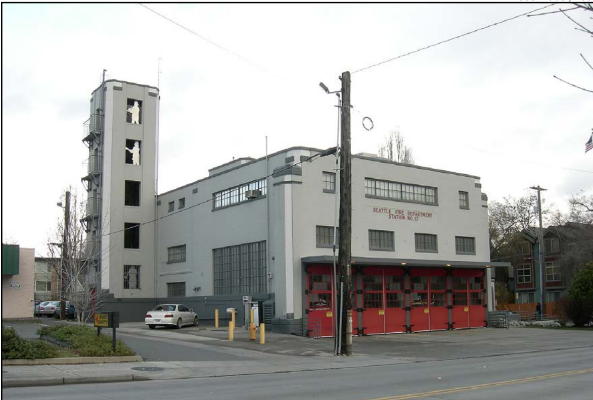
Figure 92 • Fire station #17, 101 NE 50th St (1930, architect unknown, City of Seattle Landmark)
