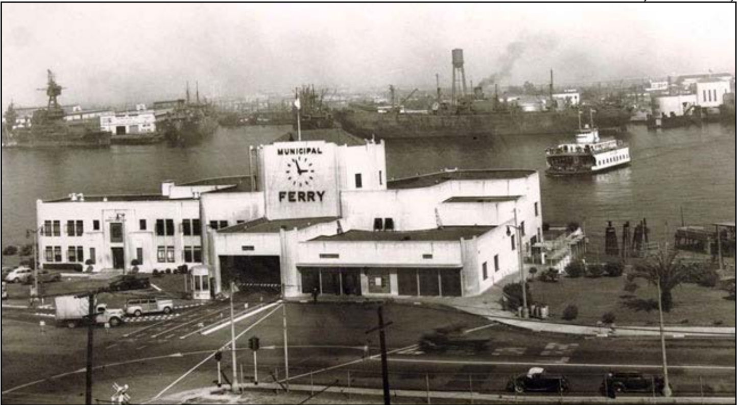
Figure 87 • San Pedro Municipal Ferry Building (1941, Derwood Lydell Irvin)
