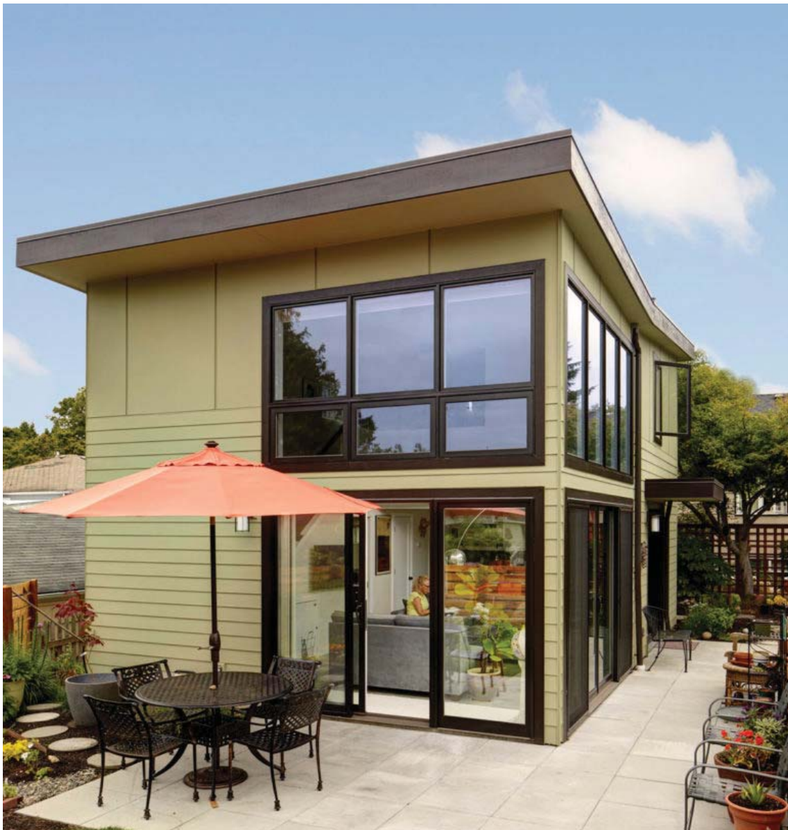
Backyard cottage designed by Nest Architecture & Design, located in West Seattle. Photo by Alex Hayden Photography, used with permission.
