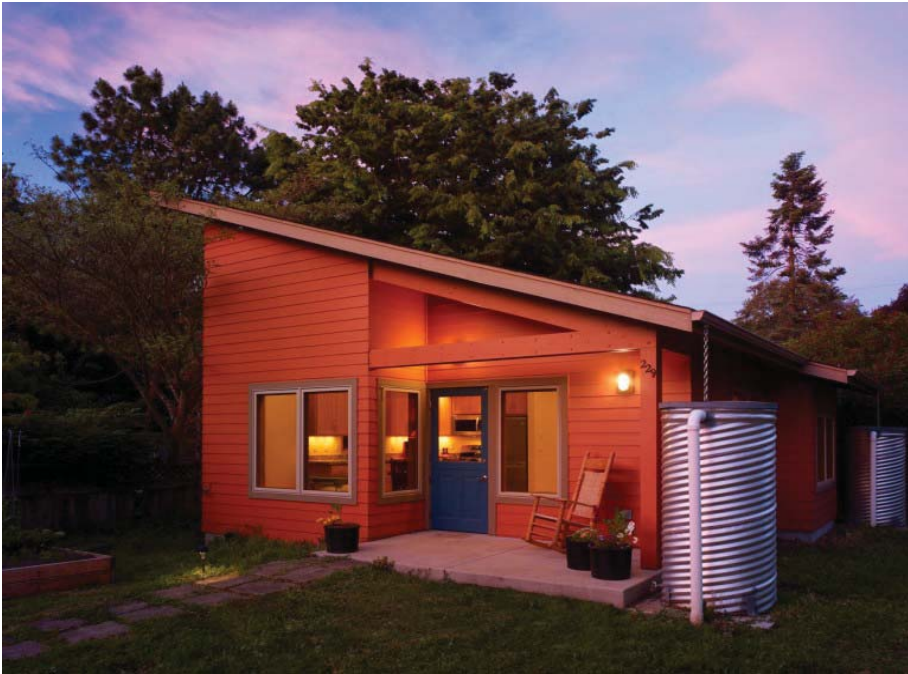
Portland ADU by Rainbow Valley Construction (Used with permission.)
