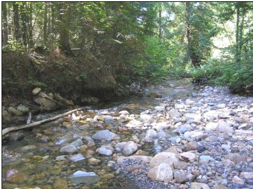
Figure 5.4-9. Channel conditions downstream of the Highway 31 culvert at Sweet Creek. Note the eroding left bank and lack of instream large woody debris.
