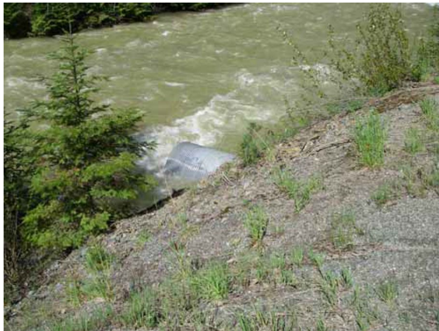
Figure 5.4-6. Outlet of culvert under Sullivan Lake Road draining NF Sullivan Creek.
