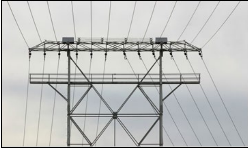
Figure 6.4 Tent covers on H-frame transmission towers
