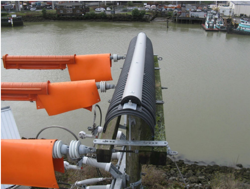
Figure 6.3 Osprey nest excluder and insulated conductor cover
