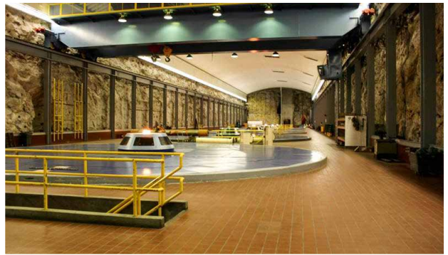
In 2015, staff repaired and returned Boundary Dam's generator unit 53 to service before the peak generation season on the Pend Oreille River in half the repair time expected and $1 million under budget. The unit went down in 2013.
