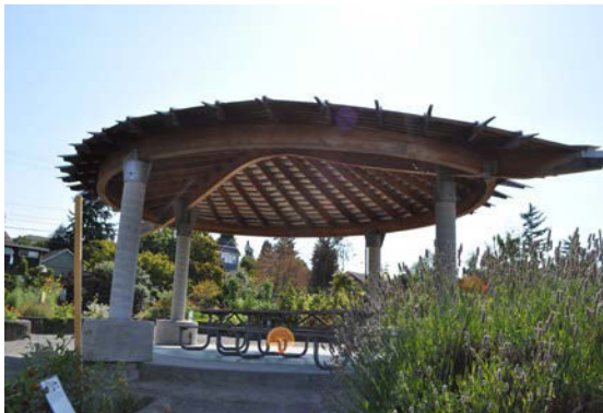
Gathering Pavillion at Bradner Gardens Park
