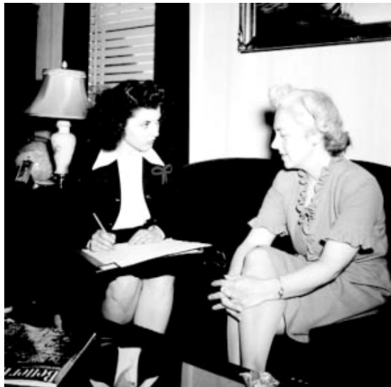
On-site traffic interview by Seattle Engineering employee, circa 1946. Neg. #40581
