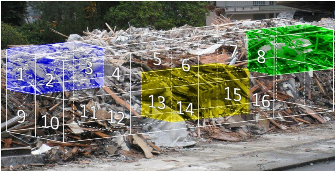
Figure 5. Visual Overlay for Direct Load Method Showing “Cells” of Material
