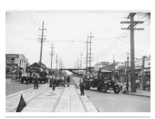
1934 pre-cast concrete slabs being set along Beacon Avenue South for the streetcar tracks. This WERA project provided work for numerous individuals in a time when work was scarce. Source: University of Washington Libraries, Special Collections, UW20653z.
