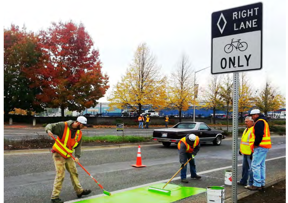
Crews painting a green bicycle lane
