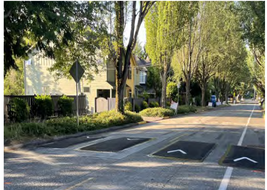
Speed cushions on 15th Ave S between Atlantic & Massachusetts help to slow traffic.
