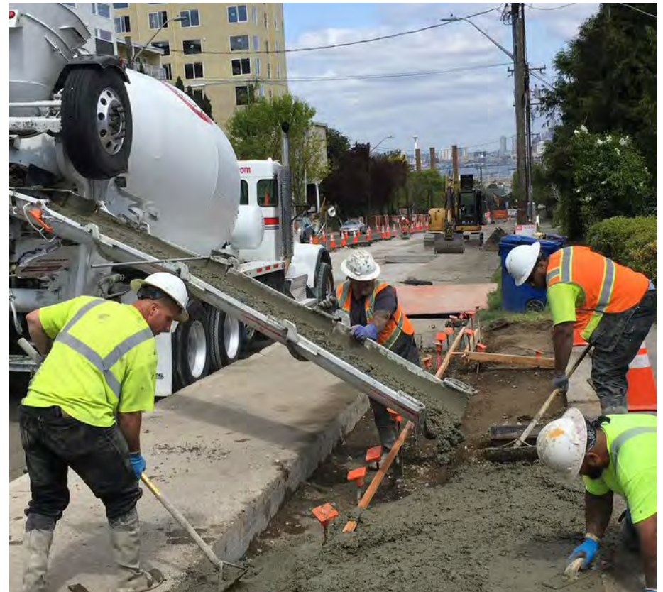
Construction crew at work in West Seattle
