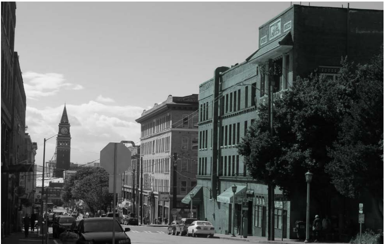
Unreinforced Masonry Buildings require significant retrofits prior to occupation above the ground floor
