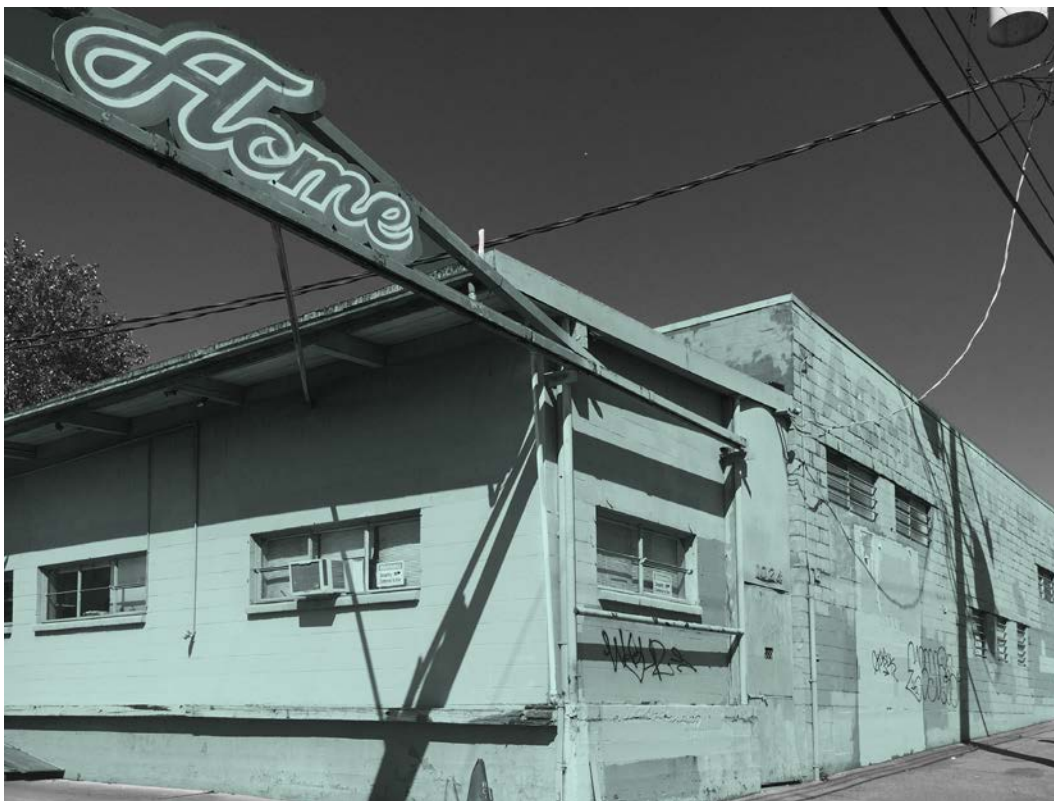
Many structures throughout the district are in need of revitalization
