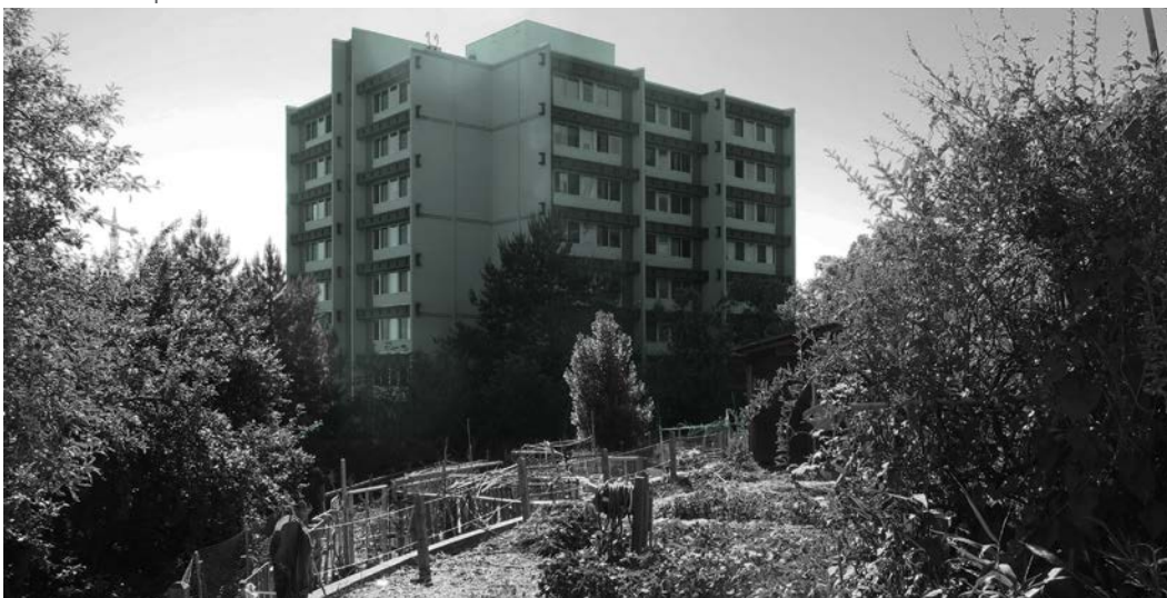
Existing affordable senior housing in the CID
