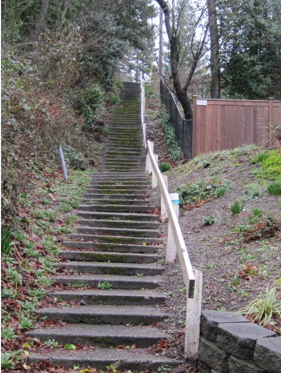
SW Holly St - First historic street car slab stairway reset and rail upgrade
