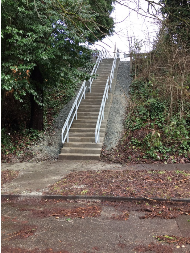
SW Holly St - First historic street car slab stairway reset and rail upgrade
