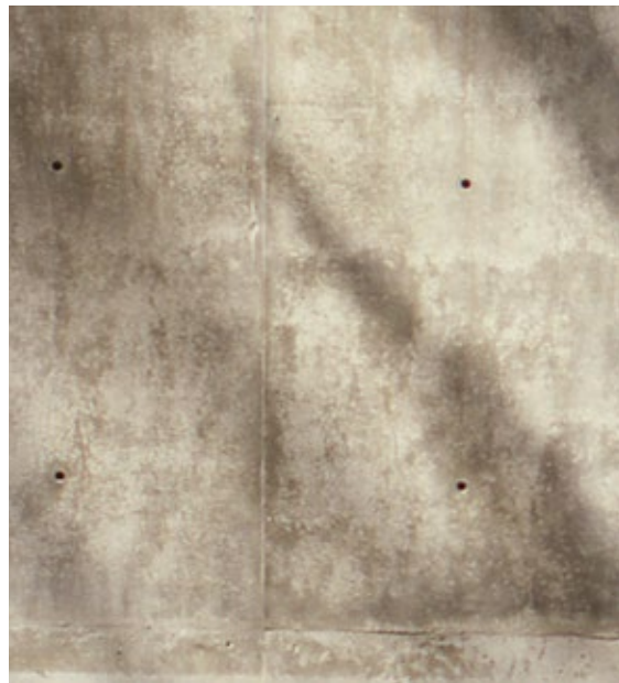
CONCRETE AT PLANTERS AND SIDEWALK
