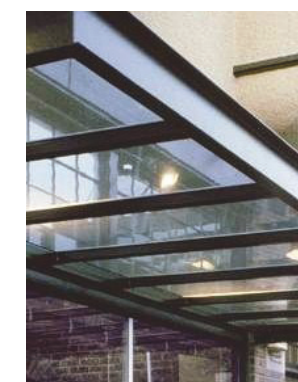
⑦ PAINTED BLACK STEEL OVERHEAD WEATHER PROTECTION
