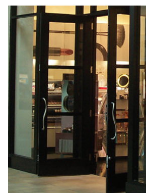
⑥ BLACK ALUMINUM STOREFRONT GLAZING SYSTEM
