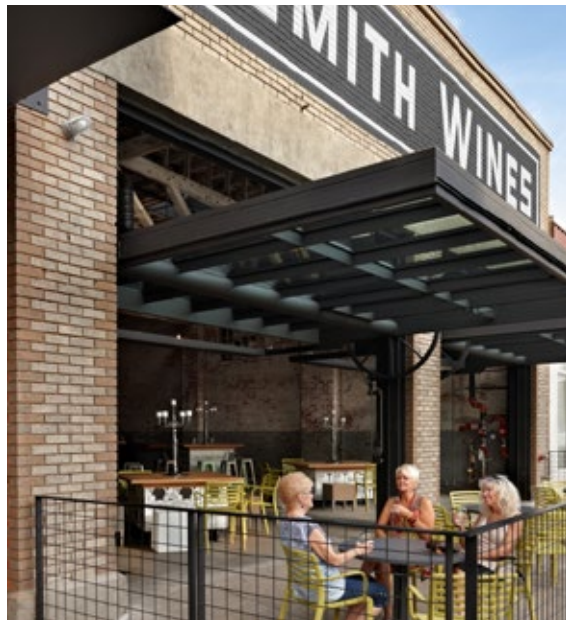
METAL AT STOREFRONT
