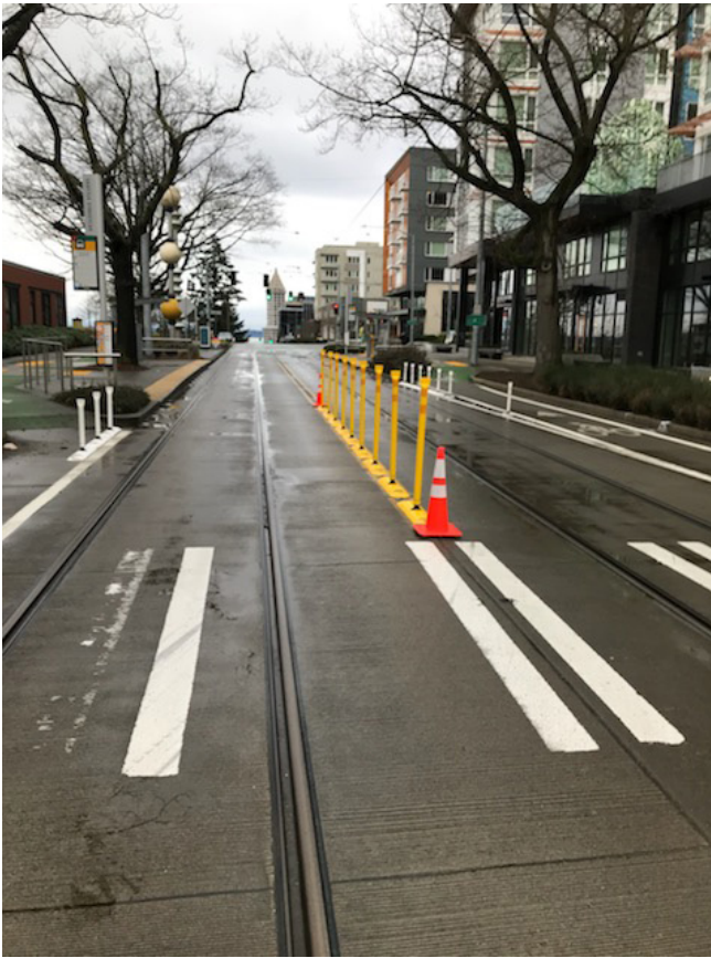
East Yesler and 10th Ave. E tuff posts
