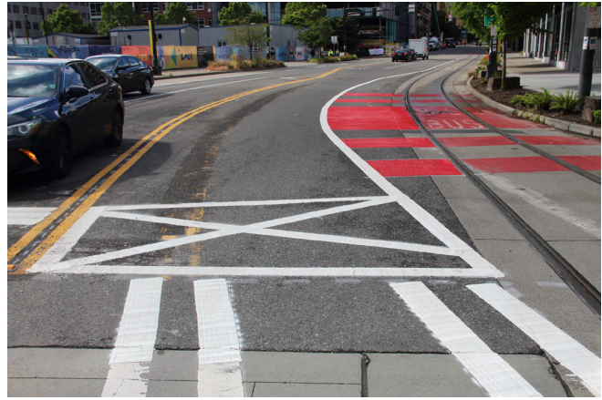
Westlake Avenue and Valley Street Re-channelized roadway
