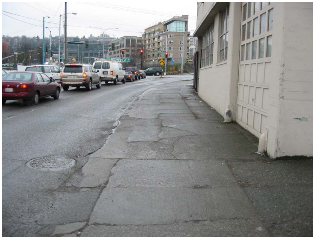
Figure 4.12 Existing Sidewalk Facilities on Mercer Street
