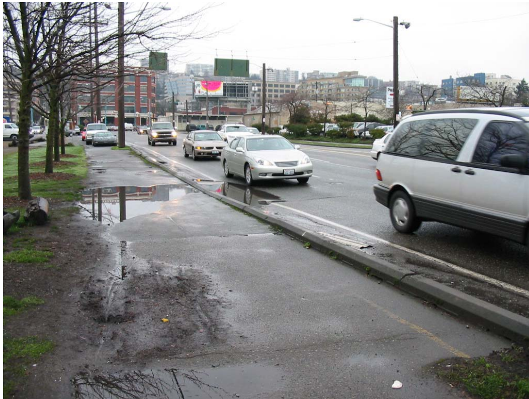
Figure 4.11 Existing Pedestrian Pathway on the North Side of Valley Street
