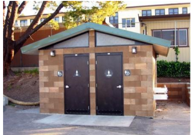
Figure 34. Pre-fabricated free-standing bathroom with exterior water fountain.
