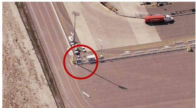
Figure 30. Typical on-terminal portable toilet location at the Port of Los Angeles.
