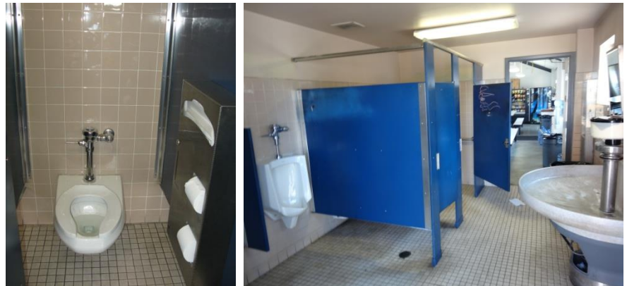
Figure 20. Bathrooms adjacent to the longshoremen (ILWU) break/lunch rooms (locations c, j, and l).
