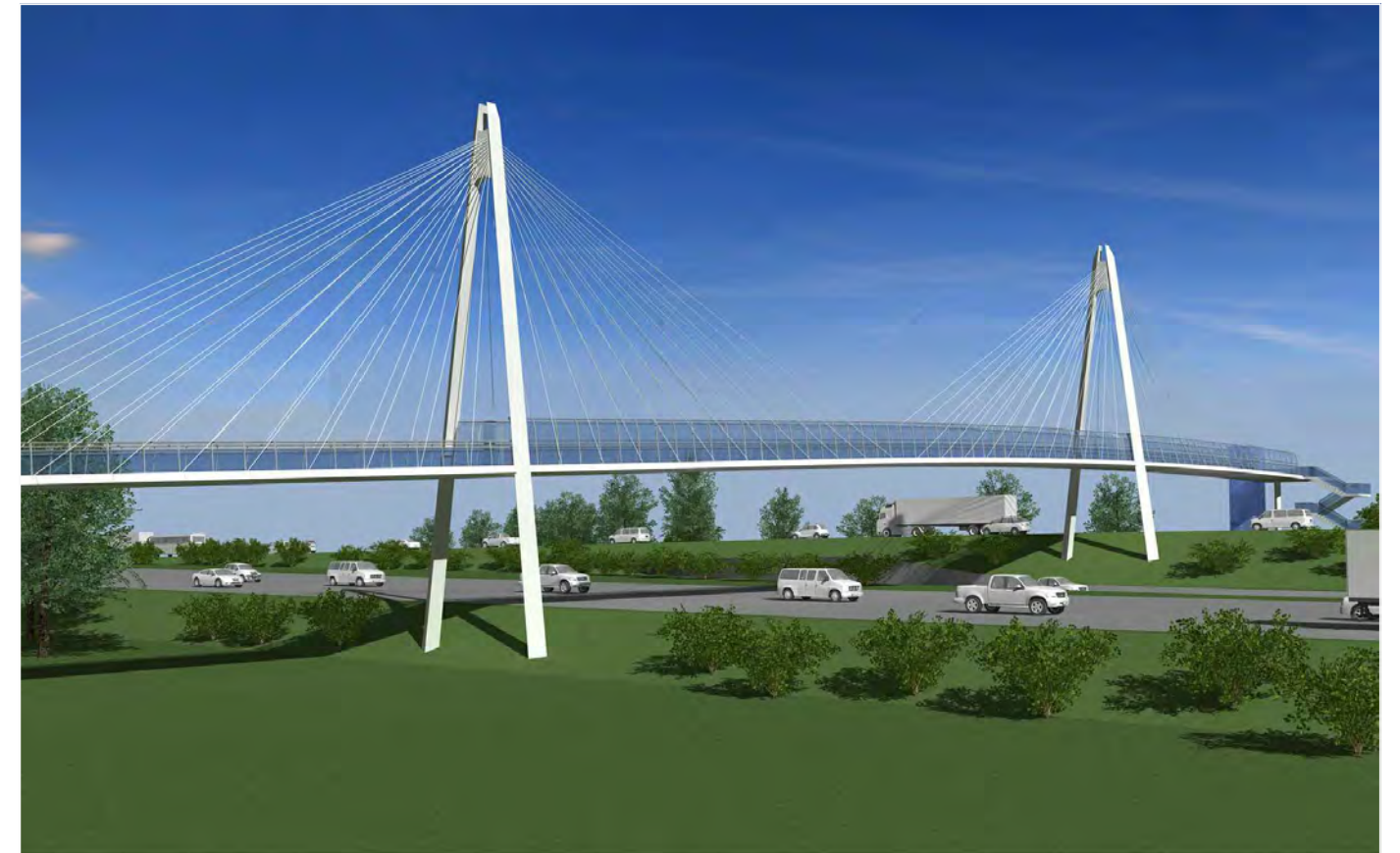
SOUTH ALIGNMENT MAIN SPAN CABLE-STAYED BRIDGE (WITH A-TYPE PYLON SHOWN)
