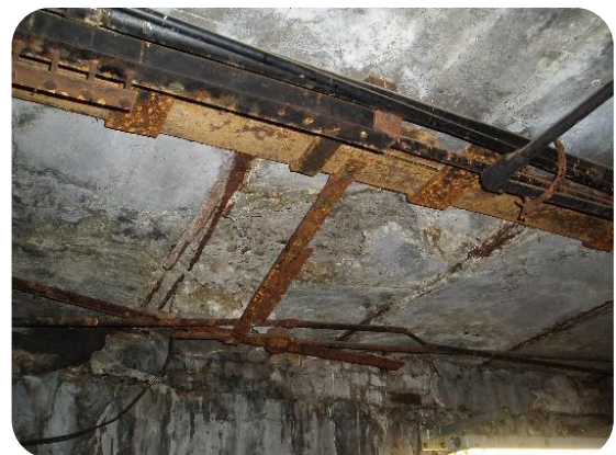
Areaway Below Sidewalk
