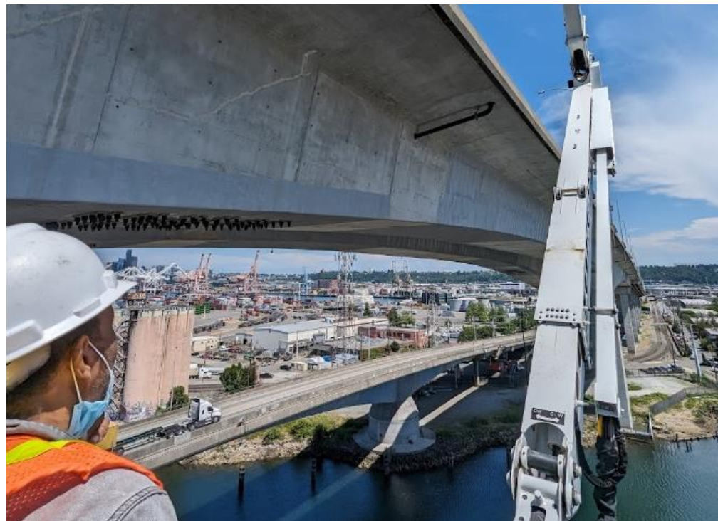
Figure 5 - June 2023 inspection of the underside of the bridge using the UBIT
