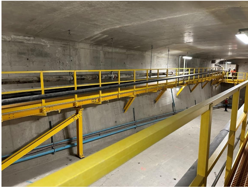
Figure 4 - New inspection platforms and lighting installed inside the bridge
