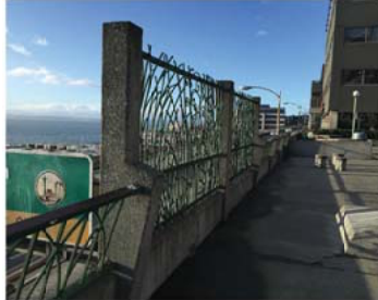
GUARDRAIL TYPE 2 (NEAR) DECORATIVE FENCE
