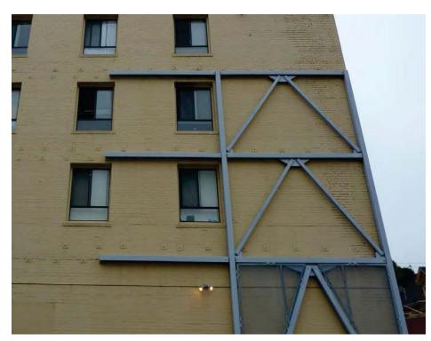
Example of seismic retrofit of masonry wall
