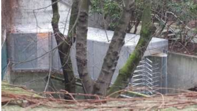
A one-way revolving door that is covered by a metal frame that leads to the garage.
