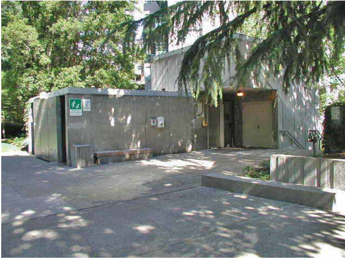
Fig. 80. Restroom facility and parking garage entrance on the right, view looking northeast, East Plaza of Freeway Park, 2005. (Photo by authors.)
