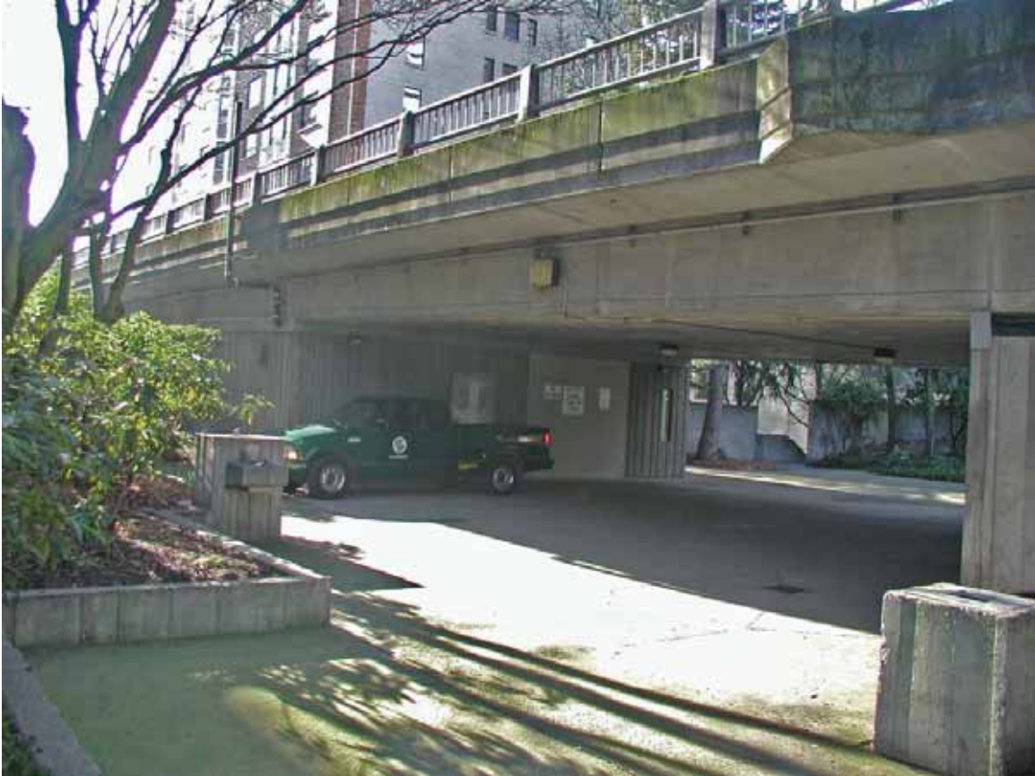
Fig. 73. Eighth Avenue overpass crew quarters, view looking southwest, Freeway Park, 2005. (Photo by authors.)
