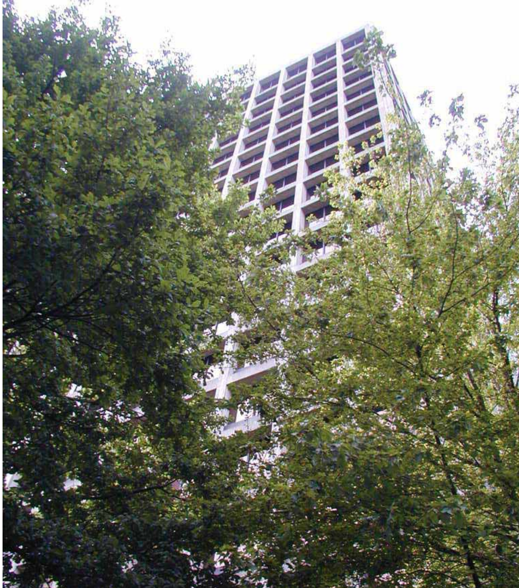
Fig. 68. View looking up at the Park Place building's southern façade from the Central Plaza, Freeway Park, 2003. (Photo by authors.)
