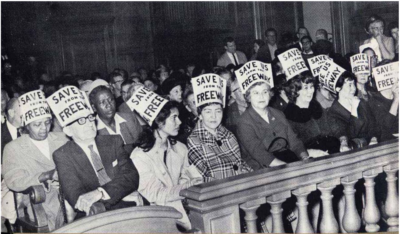
Fig. 112. Civic activists, like these in San Francisco, opposed building interstates through cities across the country. (Halprin Freeways 155.)
