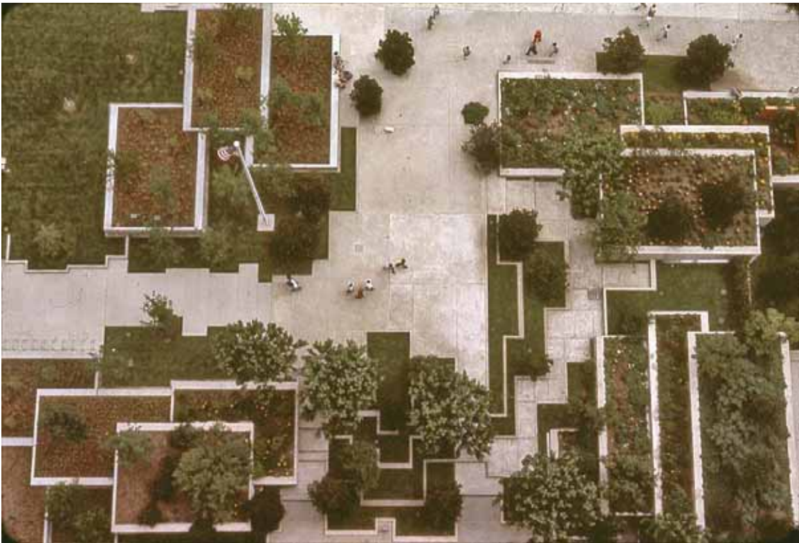
Fig. 6. Aerial view from Park Place southeast over West Plaza, Freeway Park, ca. 1976. (Danadjieva & Koenig Associates' image archive.)
