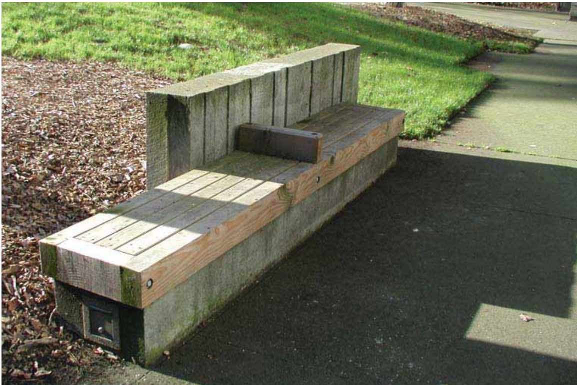
Fig. 14. Bench with replaced wood and sleep barrier, view southwest at the northeastern edge of Central Plaza, Freeway Park, 2005. (Photo by authors.)
