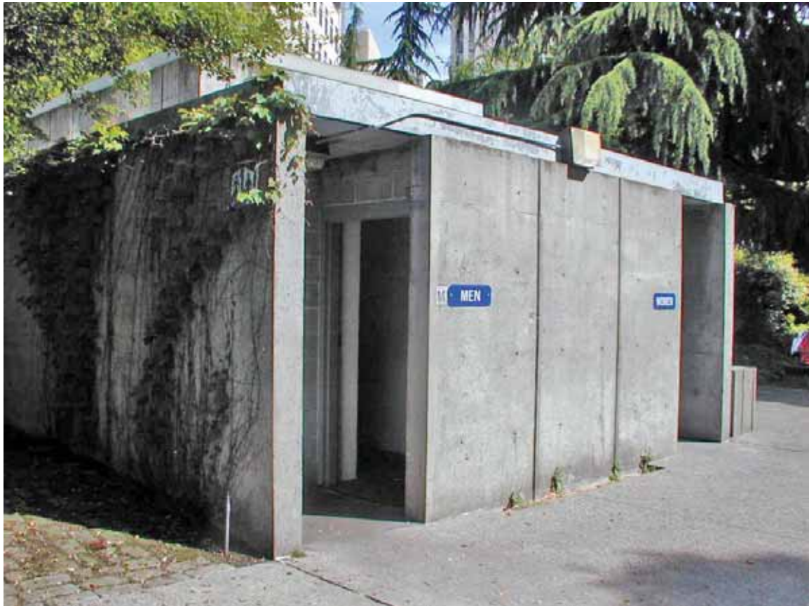
Fig. 79. Restroom facility, view looking southeast, East Plaza of Freeway Park, 2003. (Photo by authors.)
