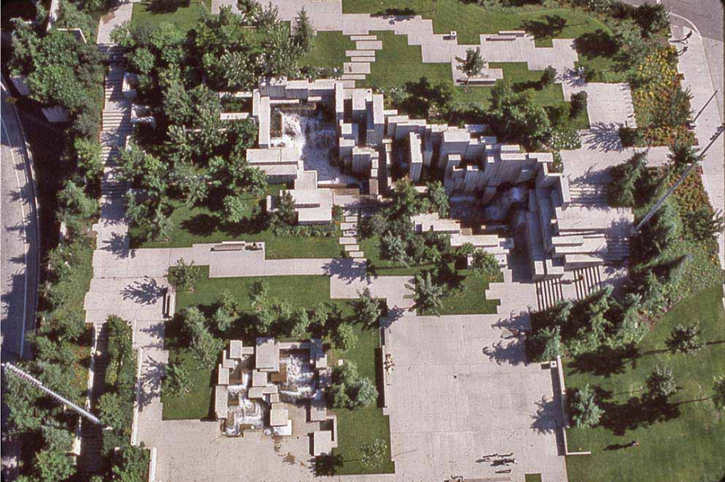
Fig. 48. Aerial view looking northeastward down from Park Place of Central Plaza, Freeway Park, ca. late 1970s or early 1980s. (Danadjieva & Koenig Associates' image archive.)
