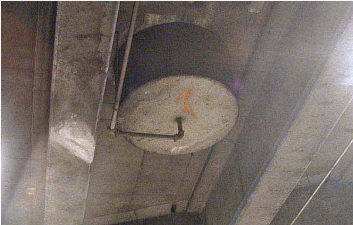
Fig. 11. Vertical tree planting tubes below Freeway Park's deck and above I-5, view upward and eastward from near the Central Plaza Canyon's pump room, Freeway Park and I-5, 2003. (Photo by authors.)
