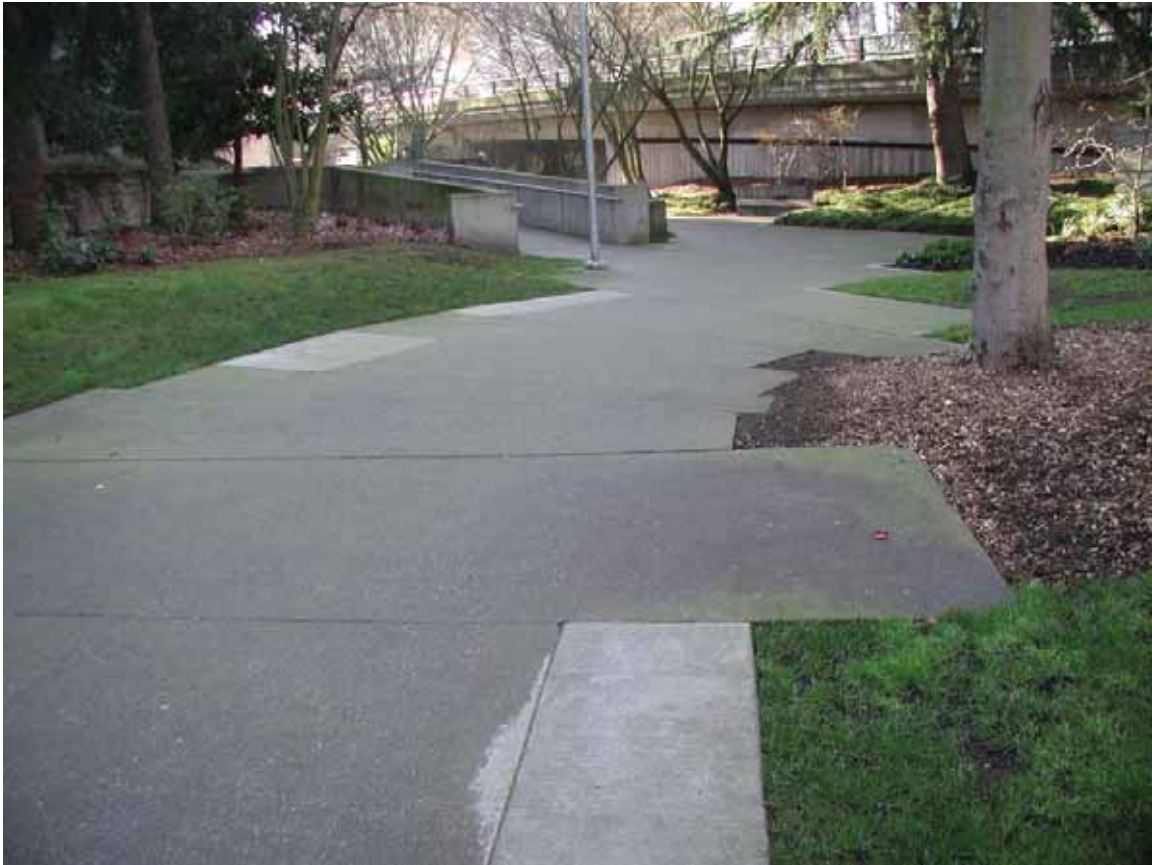
Fig. 84. New concrete pours at the East Plaza, view looking south towards the Eighth Avenue overpass, Freeway Park, 2005. (Photo by authors.)
