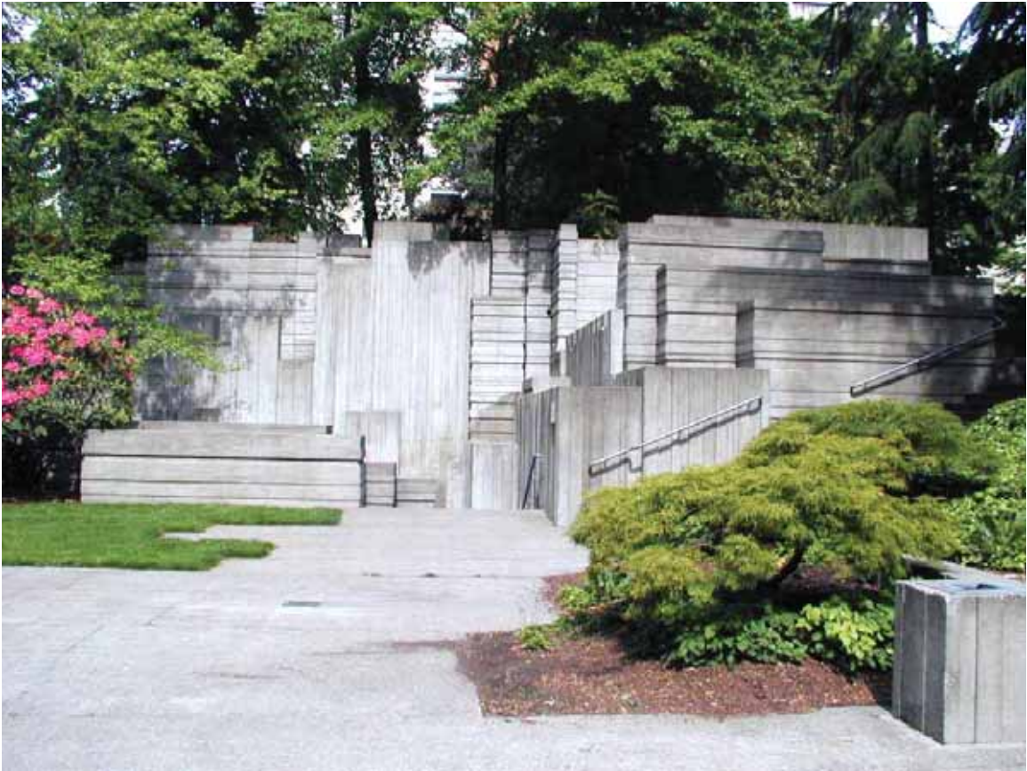
Fig. 54. Central Plaza Canyon fountain southwest facade, view northeast, Freeway Park, 2003. (Photo by authors.)
