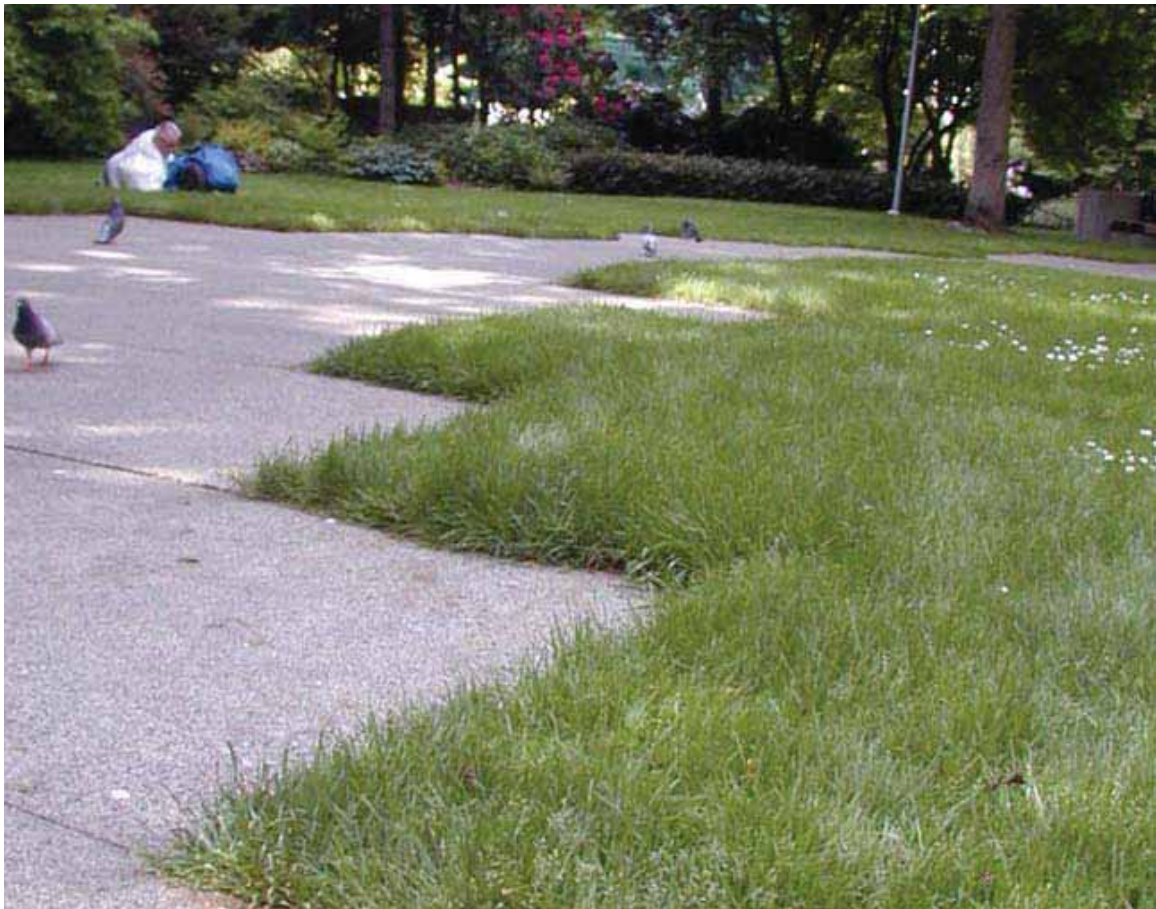
Fig. 81. Exposed aggregate path at the East Plaza, view looking south, Freeway Park, 2003. (Photo by authors.)
