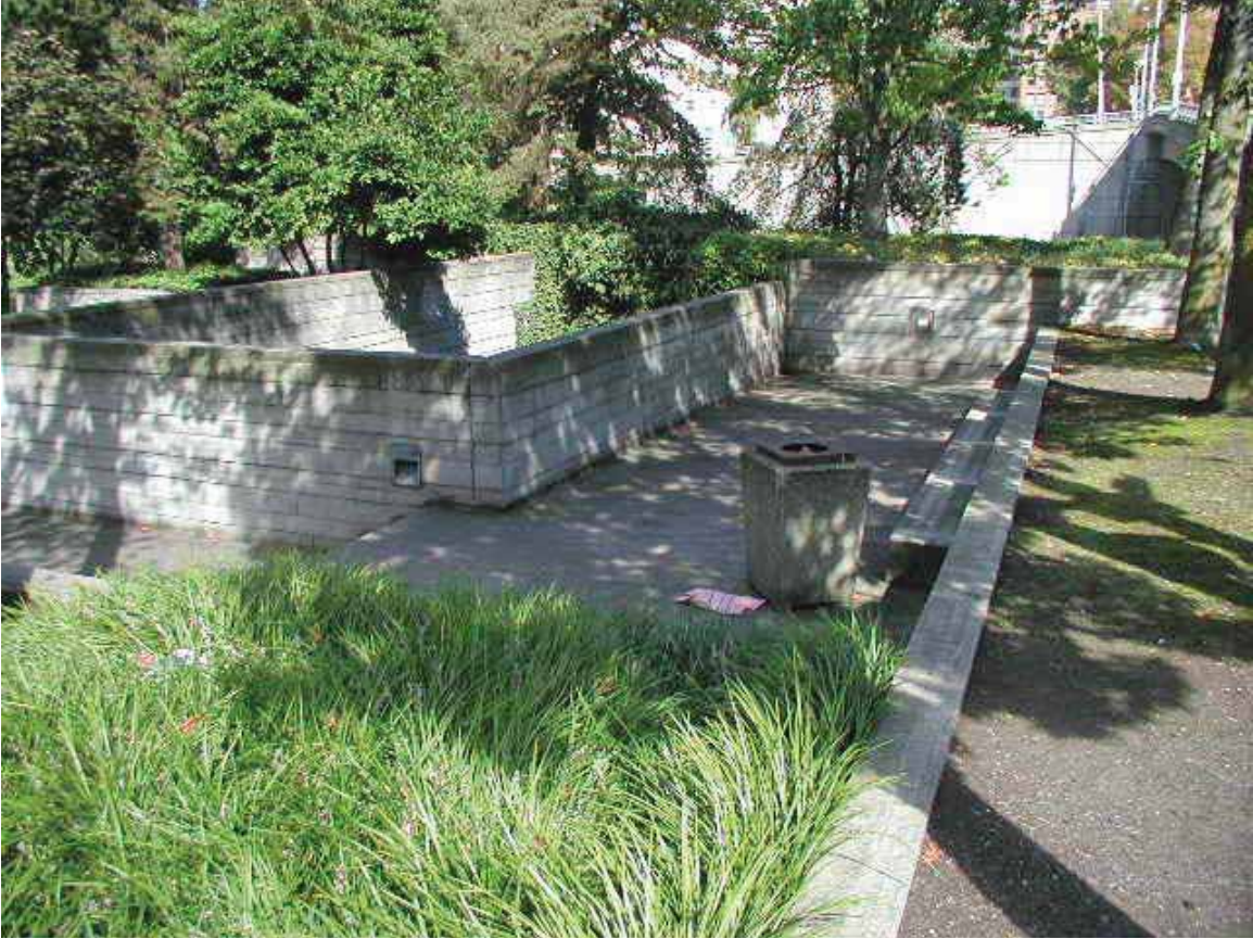
Fig. 27. Far southern seating area of Freeway Park near Spring Street with trash receptacle that is not original to the design, view looking northeast, 2005. (Photo by authors.)
