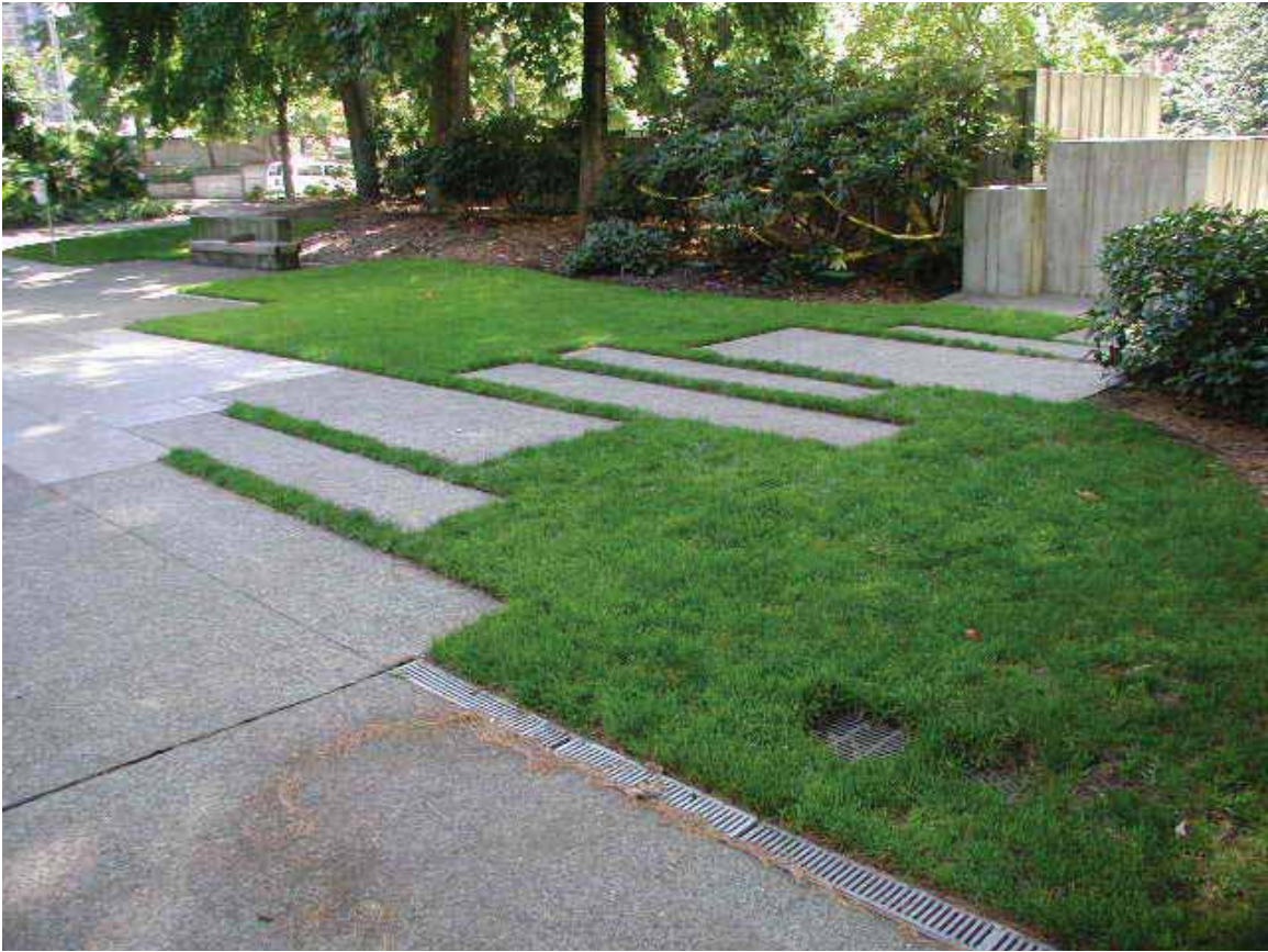
Fig. 5. Stepped concrete paths, view south at upper Central Plaza, Freeway Park, 2005. (Photo by authors.)
