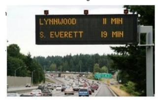
Photo 7. DMS installed along I-5 in Seattle
